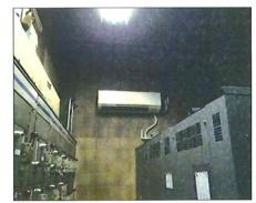
Condensate Drain Over Electrical Gear
