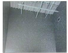
Steel Joist and Metal Deck Construction
