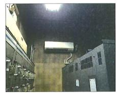
Condensate Drain Over Electrical Gear
